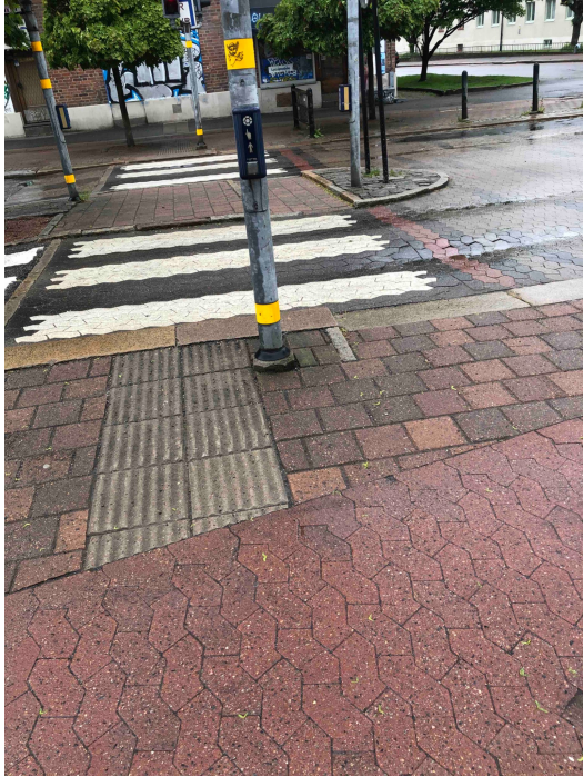
Picture 24. Textured surfaces for people with visual impairments, posing an obstacle to wheelchairs. To the right side is a bevelled kerb for wheelchairs. Photo: Jörgen Lundälv
