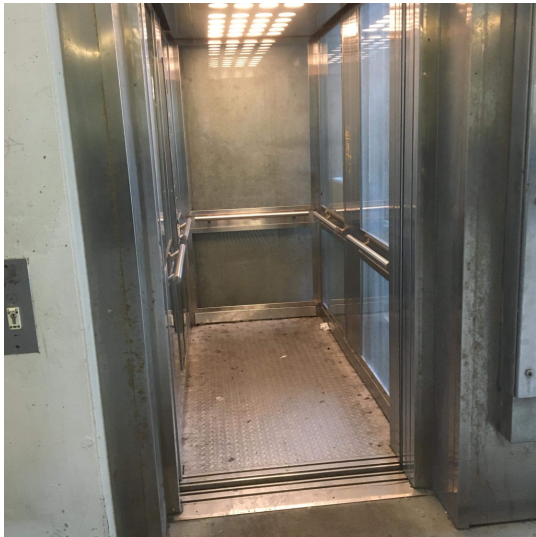
Picture 27. Uncleaned and foul-smelling lift area. Photo: Per Olof Larsson
