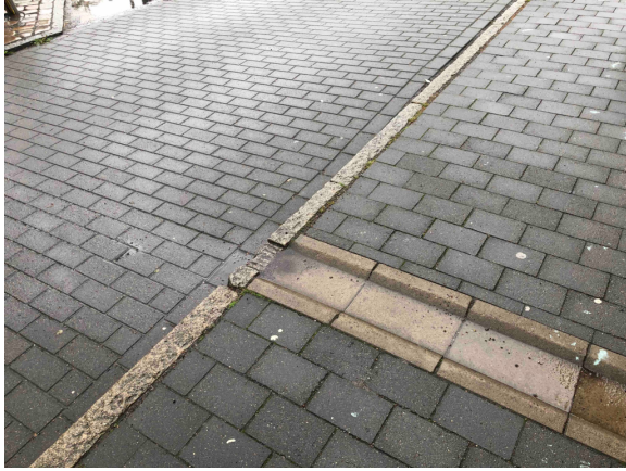
Picture 22. Barriers to wheelchairs in the street environment, with level differences. Photo: Jörgen Lundälv
