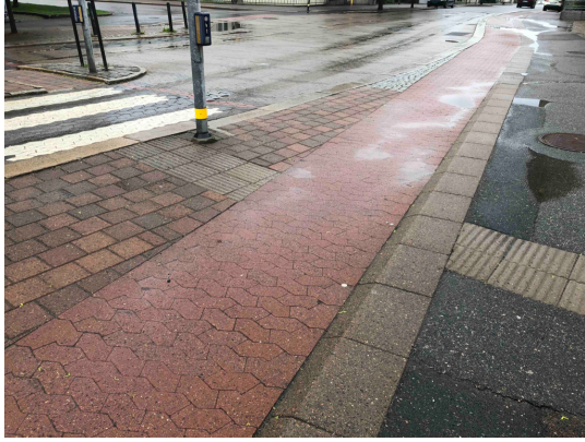
Picture 26. Wheelchairs, prams and cyclists have to compromise on space. Level difference up towards pavement. Photo: Jörgen Lundälv
